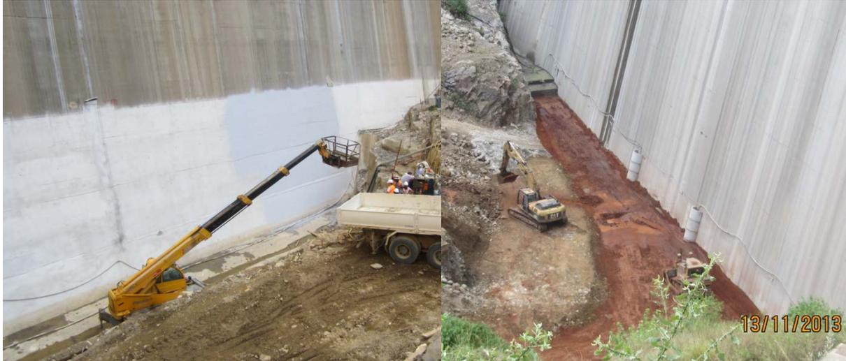
*Fig.4 Application of sprayed membrane and clay backfilling*
