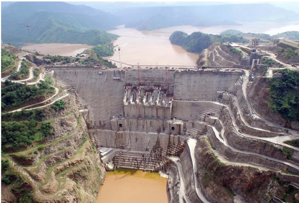
*Fig.1 - Gibe III dam nearing completion while impounding the reservoir*
