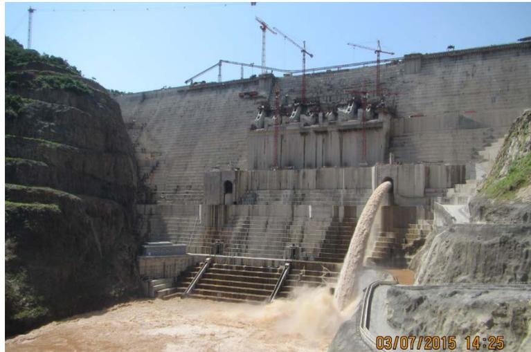
Fig. 6 Wet Commissioning of Left Middle Level Outlet ( $Q \approx 300 \text{ m}^3/\text{s}$ )
