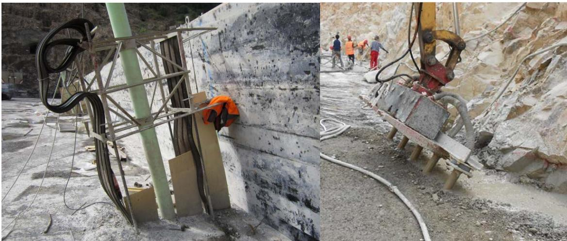
*Fig.5 RCC placement: upstream water-stops installation and GEVRCC vibration against rock.*
