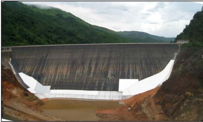
Figure 16: PVC membrane installed on the dam face.
