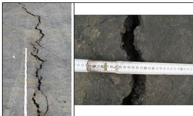
Figure 15: Open cracks on the bituminous asphalt layer exposed after reservoir drawdown
