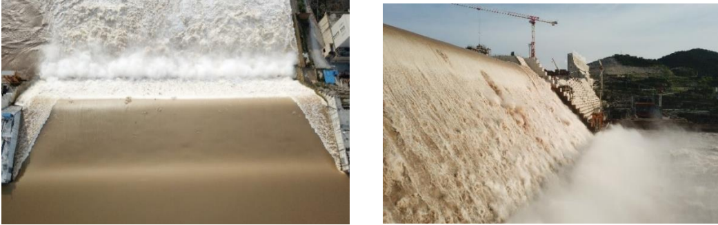
Figure 6 – GERD, Temporary Stepped Spillway with sill at 560 m asl (September 1 st , 2020).
