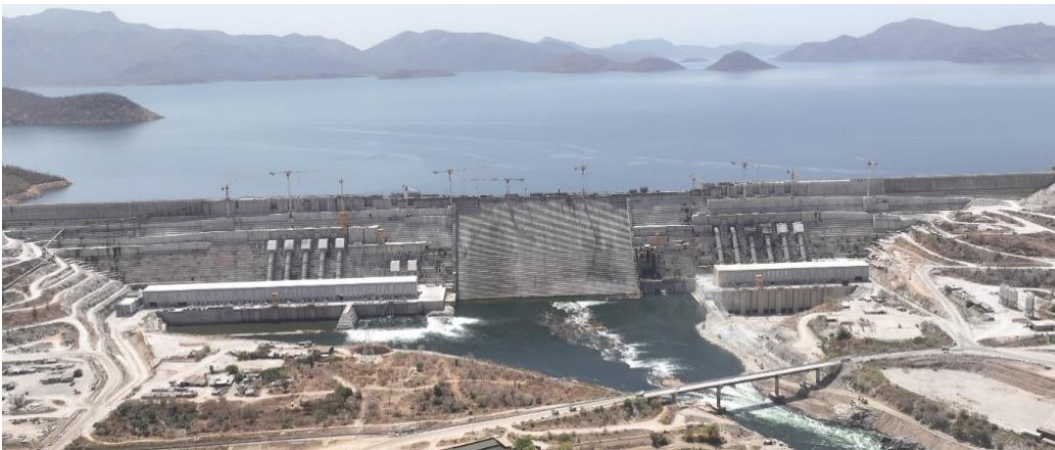
Figure 1. GERD Main Dam and powerhouses, downstream view
